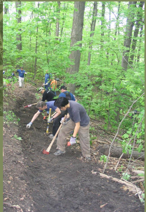
New Trail Construction
